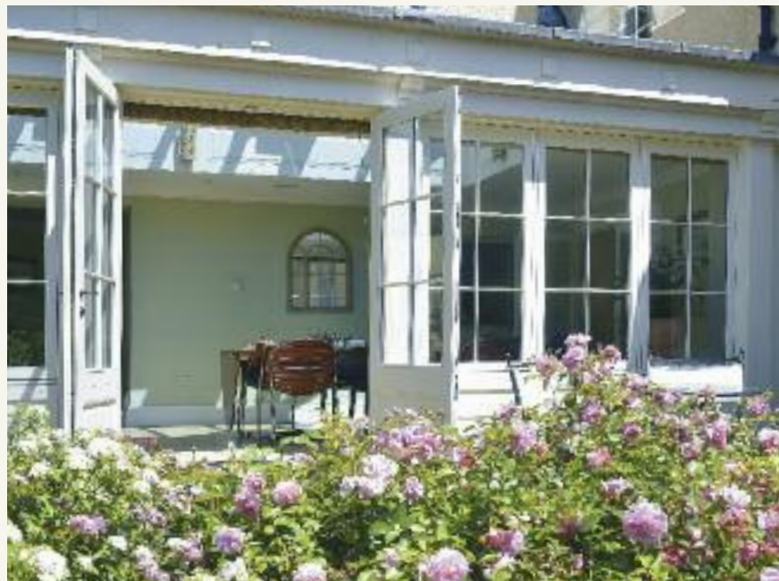
French door sets and flush casement windows, all with 18mm astragal glazing bars and finished in a colour complementary to Farrow & Ball 'White Tie'.
