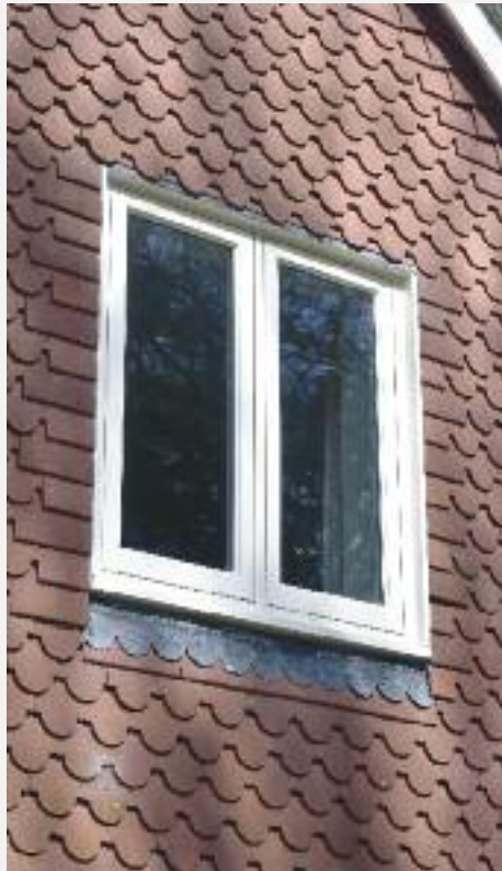
Contemporary flush casement windows, finished in 'Cream', featuring 316 coastal grade stainless steel window fastener and manufactured in Engineered European Redwood.
