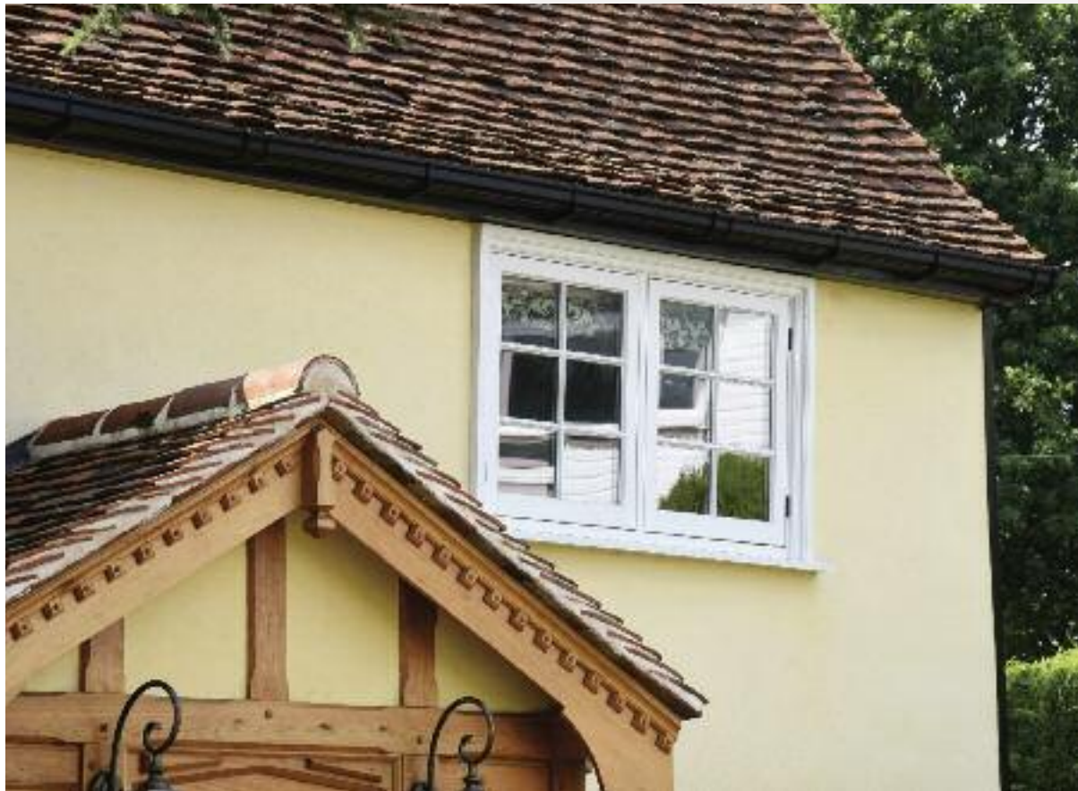
Flush casement windows finished in 'White', with 27mm astragal glazing bars and manufactured in Engineered Meranti Hardwood.
