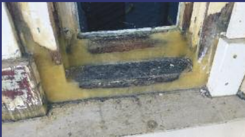
A combination of window repairs taken to extreme levels!
