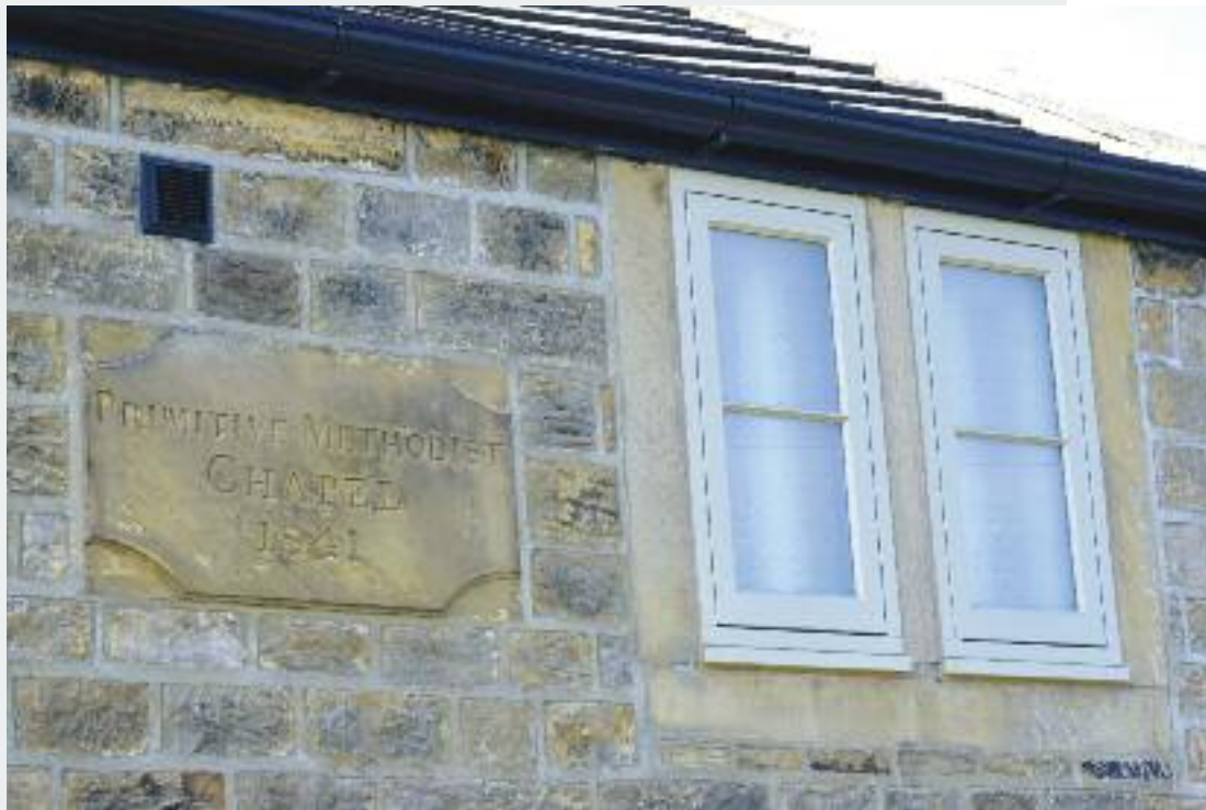
Flush casement windows in 'French Grey' with 18mm astragal glazing bars, manufactured in Engineered European Redwood.
