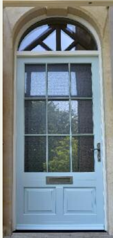
Bardwell entrance door with arched toplight, finished in a colour complementary to Fired Earth 'Nordic Light' and a 'White' frame. The door features 'Canterbury' patterned glass, 18mm astragal glazing bars and a traditional Pewter Blacksmith letter plate. Door handle sourced separately by the customer.
