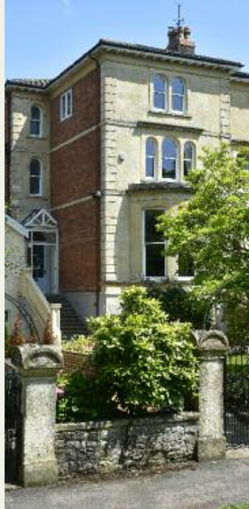
A mixture of traditional and swept head slim sash windows finished in White, with decorative sash horns and manufactured in Engineered European Redwood.
